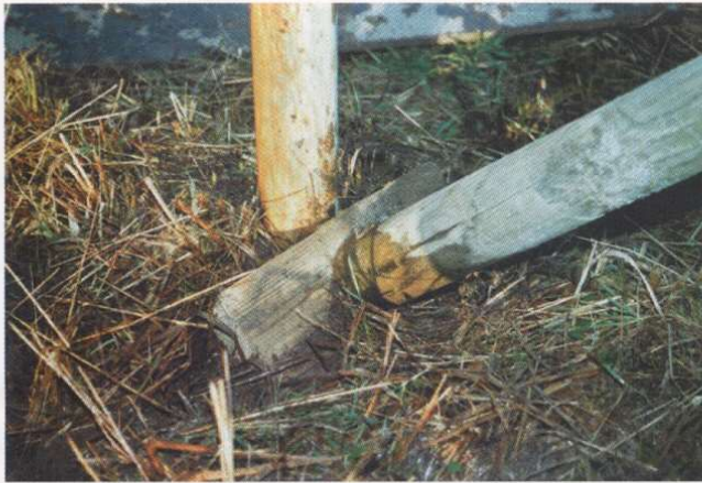
This (dx-04) shows the thrust plate with the stay placed on top
