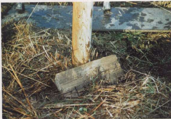
This picture shows the 'Thrust plate' in position'
